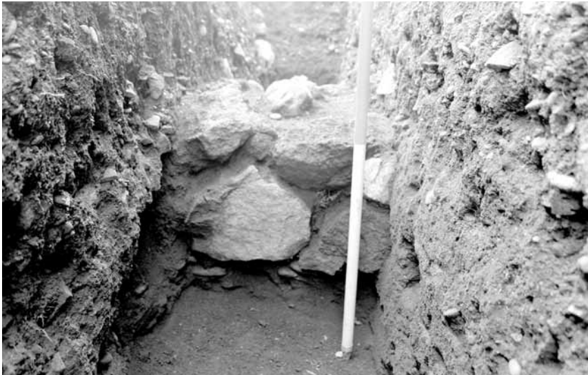
Fig. 8. Gonio. Foundation of wall A (view from the east) (A. Trzop-Szczypiorska).
