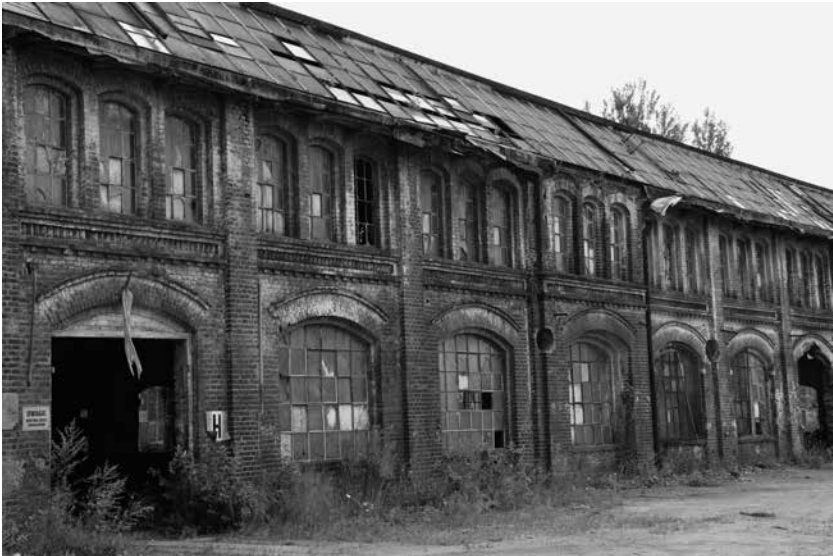
Prussian shipyard halls, Gdańsk Shipyard. Photos courtesy of John Mullen
