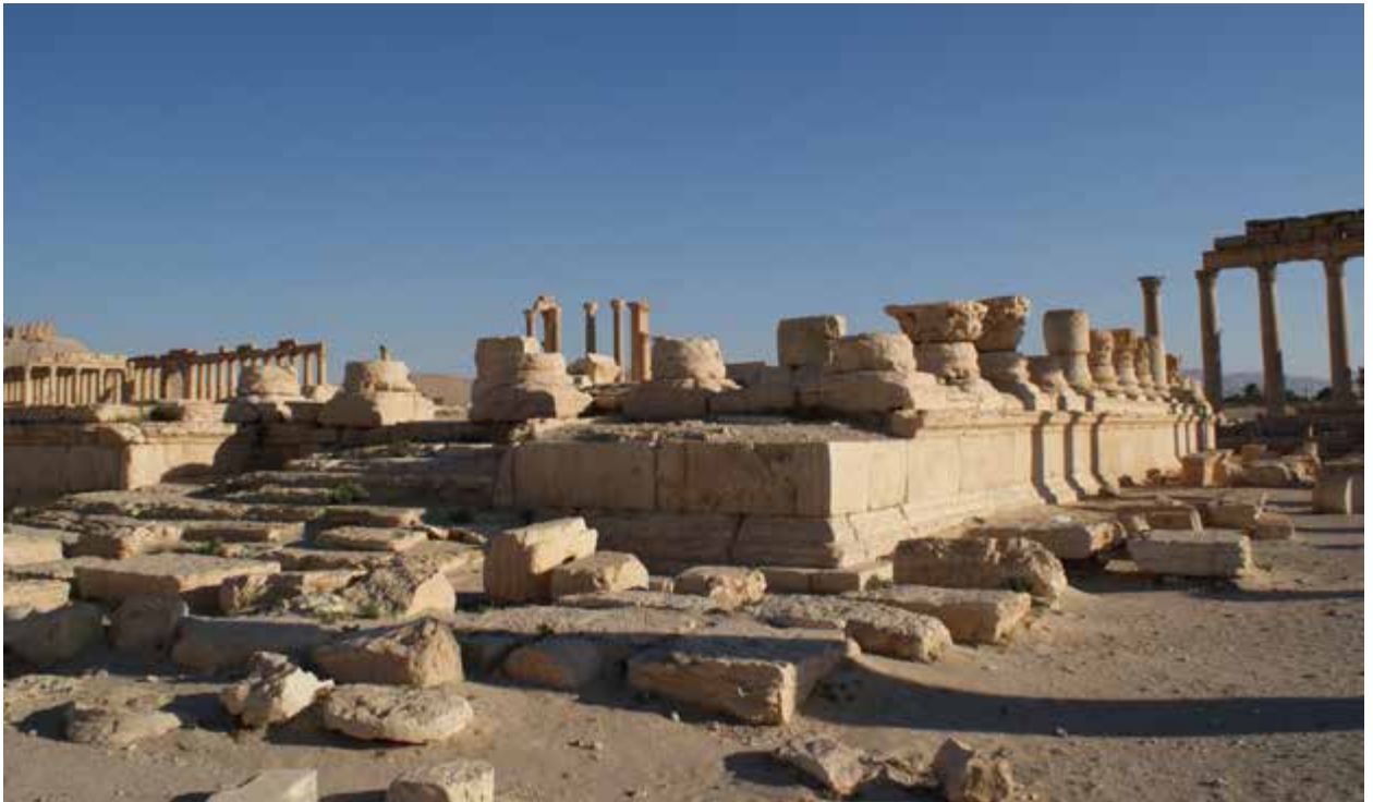
Fig. 6 The temple of Nabu (see Fig.1 No. 4), view from the south-west (photo: K. Jakubiak).
